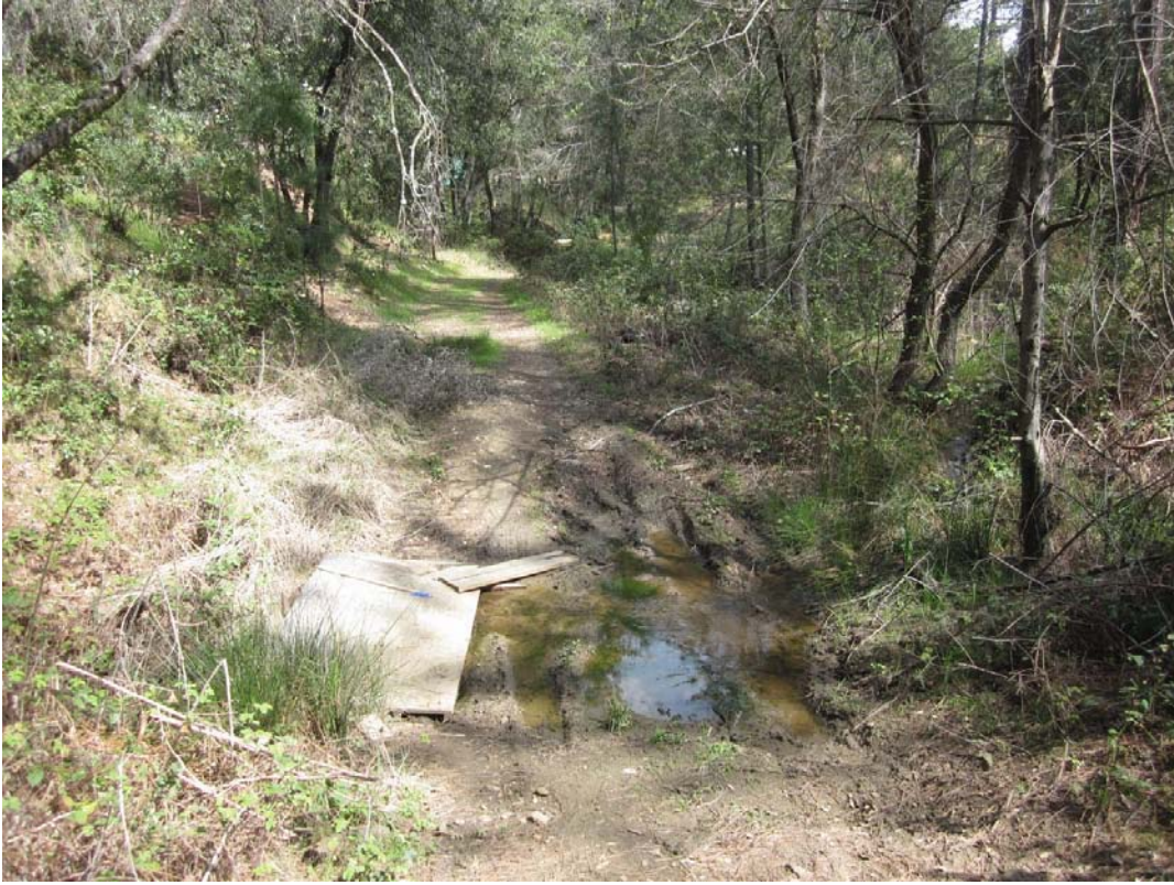
Figure 4: Access road at lower stream crossing (ford). Looking southeast.
