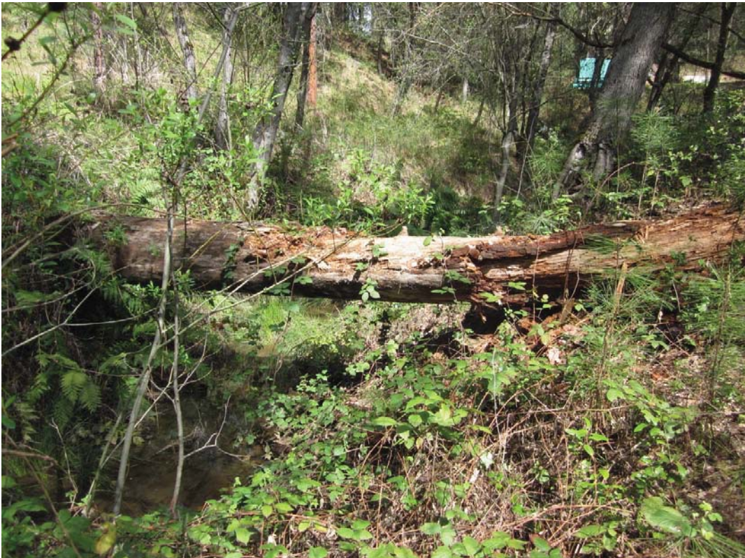
Figure 2: Looking upstream at upper access road stream crossing.
