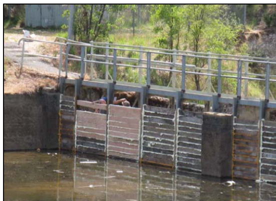
Photo 3.1-2. Flashboards being installed at the Spillway weir in 2008. The lake level will rise to the top of the flashboards, which is equivalent to the Ordinary Summer Lake Level (Photo from PLTF, 2010a).
