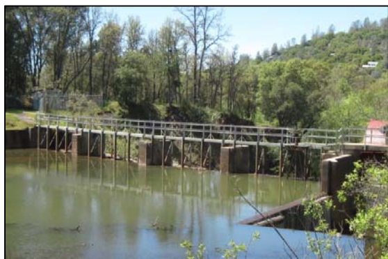
Photo 3.1-3. Spillway weir without flashboards in place, which is equivalent to the Ordinary Winter Lake Level.
