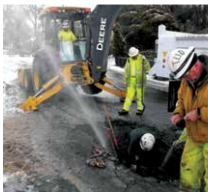
Main Line Water Break - Willow Springs
